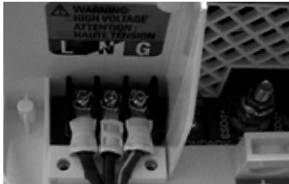
2. Connections – Using ring or captive spade connections and the proper crimping tool, attach the Line – Neutral – Ground to the appropriate terminals on the charger (Note: Label above AC connector is color coded to ensure proper installation). Repeat this procedure for the breaker side of the install. Support cable every 18" and protect from sharp edges and chafing when passing through bulkheads, and other openings all according to ABYC E-11.
